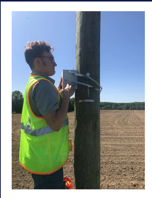
2023 Intern, Jacob Hodge installing a radar counter
